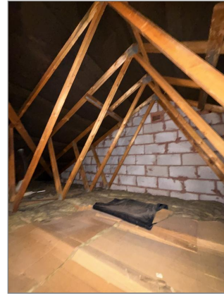
Photo - 6 Roof space
