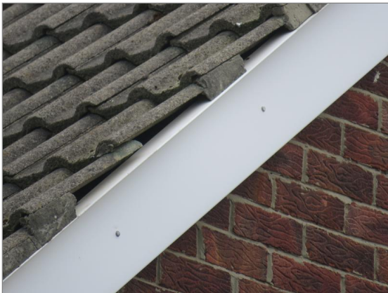
Photo - 5 Verge mortar
