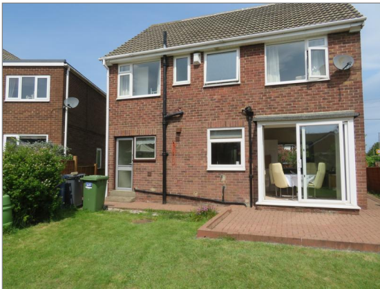
Photo - 7 Rear elevation
