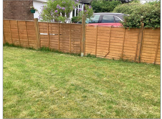
Photo - 19 Timber fencing
