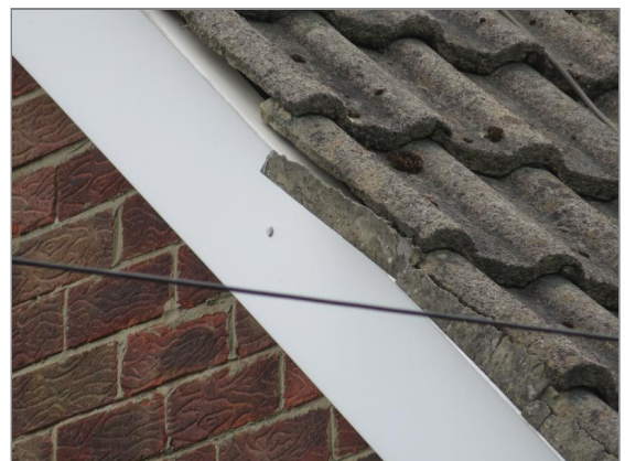
Photo - 4 Verge mortar
