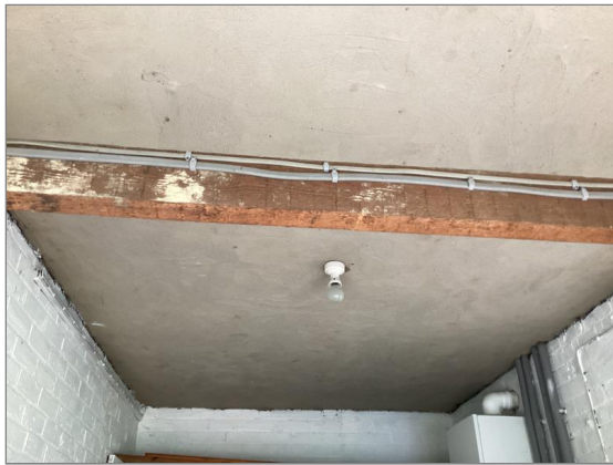
Photo - 16 Garage ceiling
